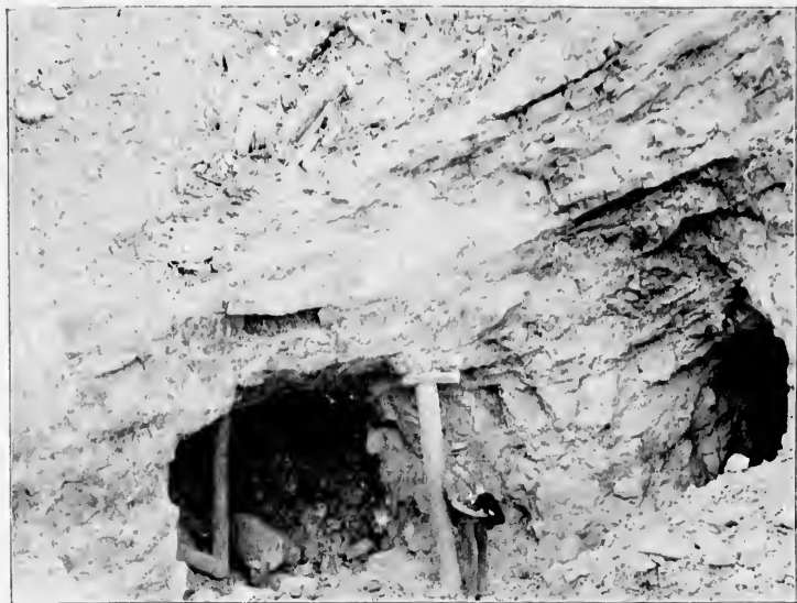
FIG. 131.—Open cut, showing the pay-streak, at Mercur, Utah. From a photograph by P. K. Hudson, 1898.
